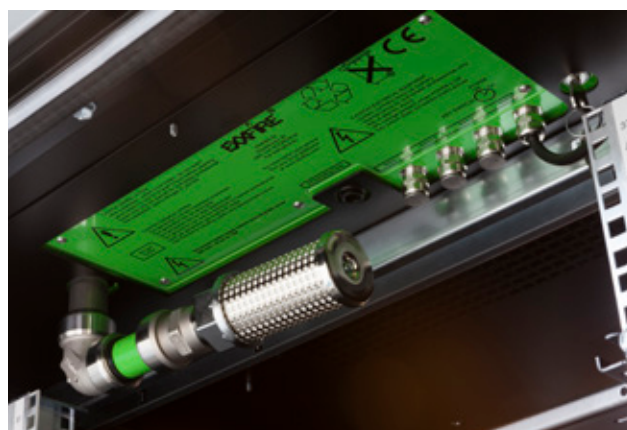
MiniCube 3,5 kW – Advanced with ExxFire fire suppression system
